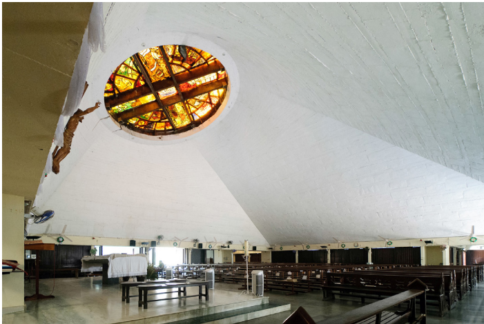
Fig. 18. Charles Correa, Salvação Church (Our Lady of Salvation), Dadar (Bombay), 1974-77 y 1983-85.
