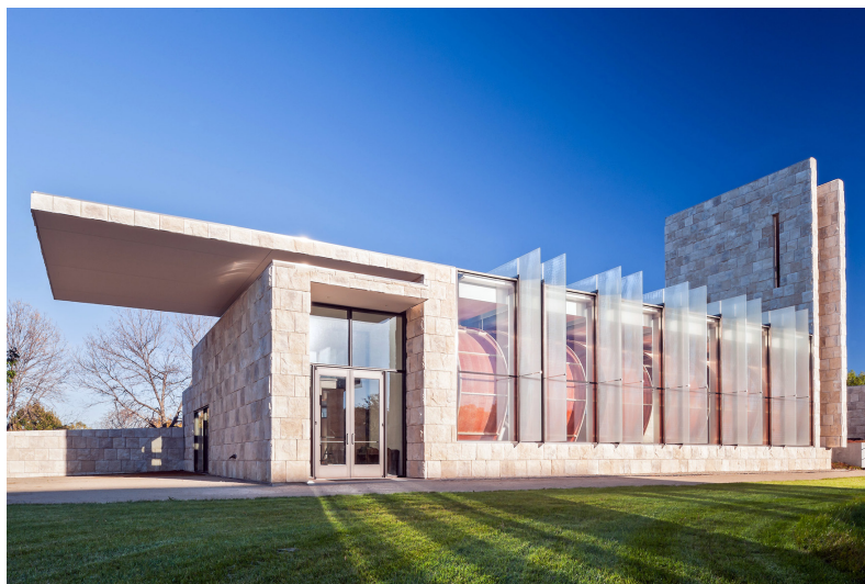
Fig. 02. HGA architects. Bigelow Chapel, United Theological Seminary, New Brighton (MN, USA); exterior.
