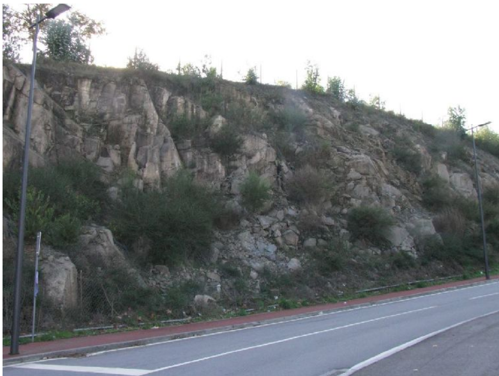
Fig. 5. Example of revegetation of a granite road slope with less than five years in Braga (Northern Portugal).
