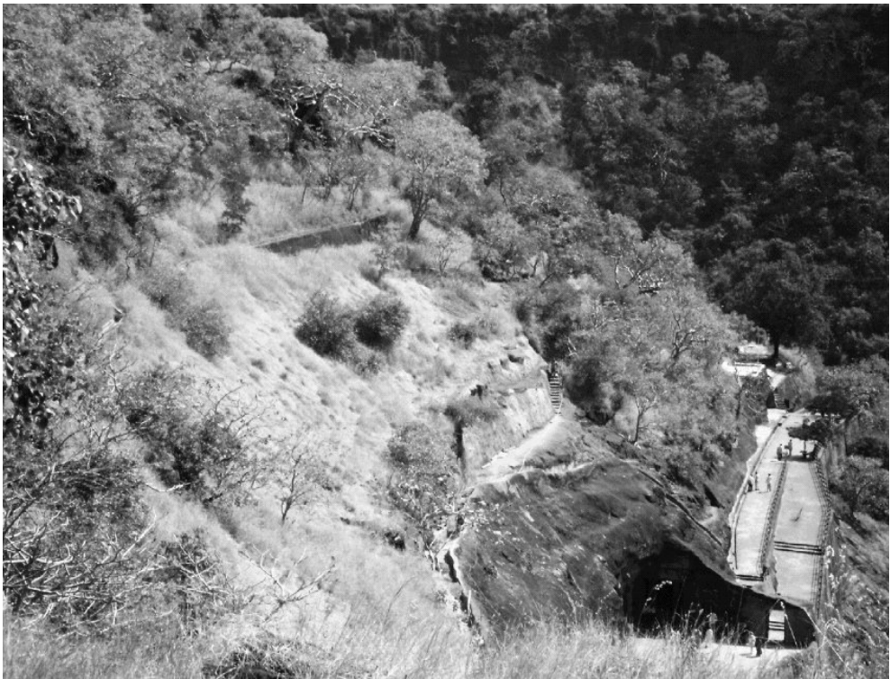
Fig. 4. Structure erected for slope protection at the Ajanta Caves World Heritage Site. It is designed “ideally” to avoid distraction of visitors’ attention from the site itself, this structure looks similarly to authentic natural (basalts) and artificial (caves) features.
